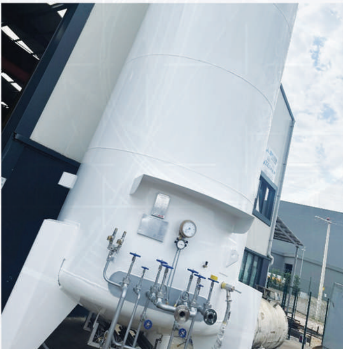
Valve group siphon design with outlet from lower grenade
